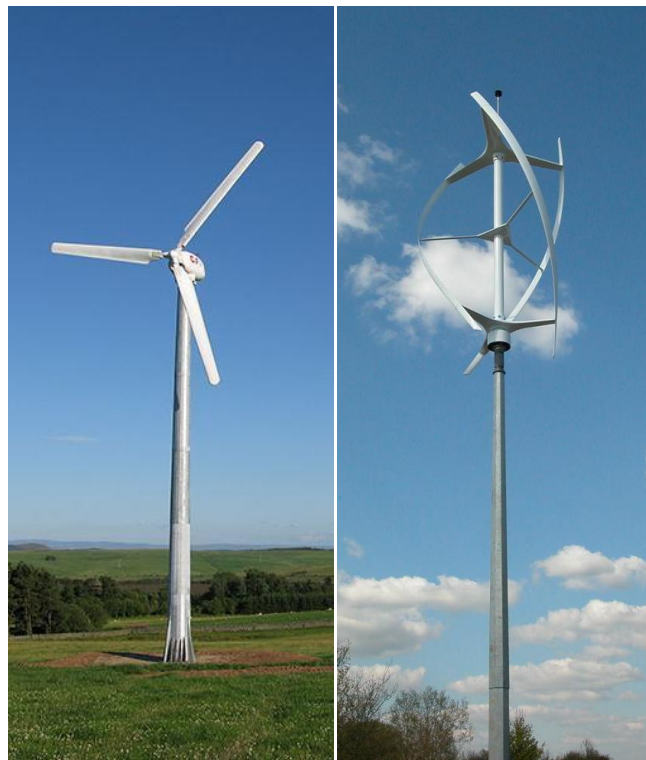
Figure 3.1: Examples of horizontal axis (left) and vertical axis (right) format wind turbines (image sources: C&F Green Energy (2015) (left), VWT Power (2014) (right))
