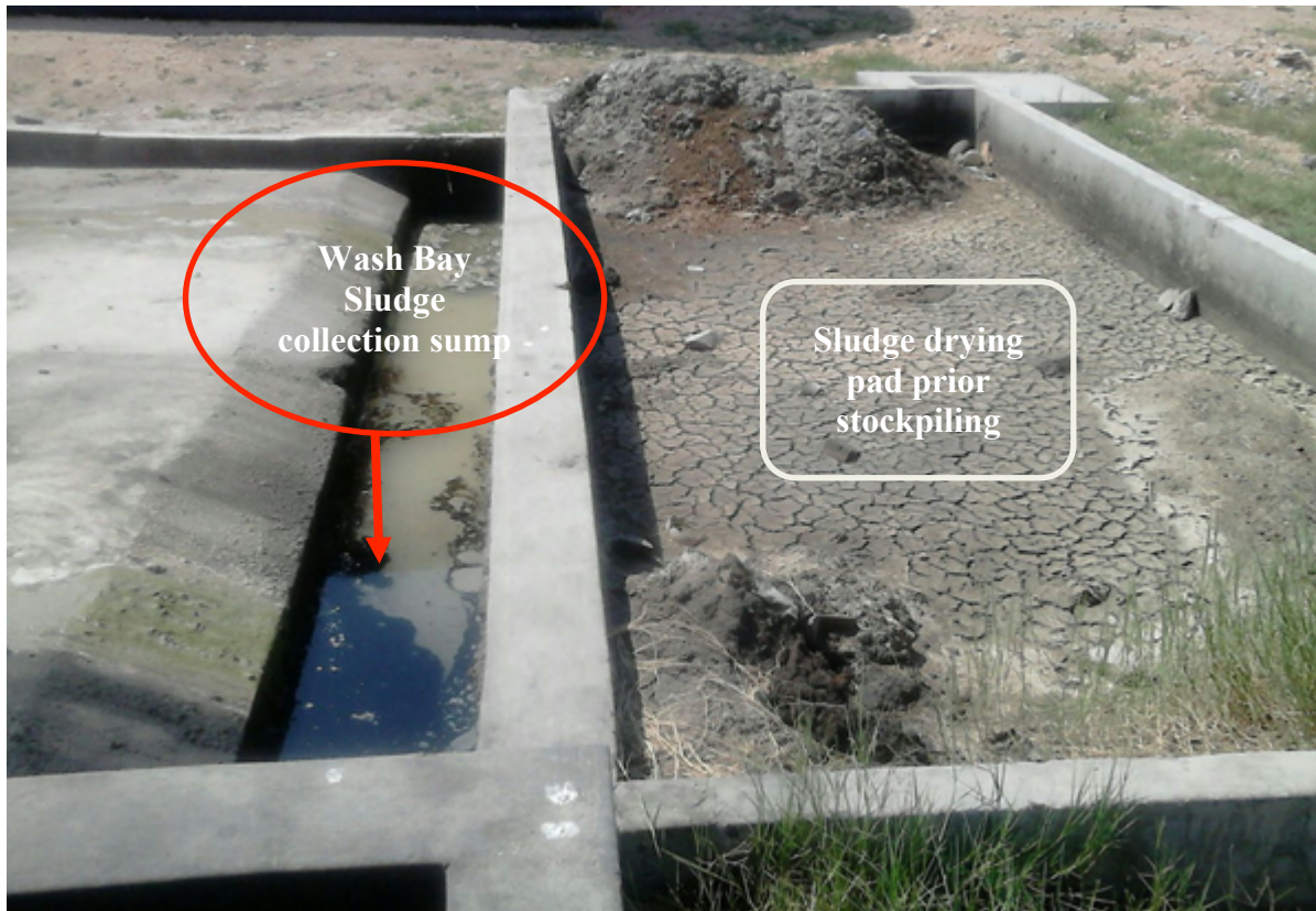
Figure 4 -Small wash bay showing recently deposited oil contaminated soils where systematic grid sampling method was applied.
