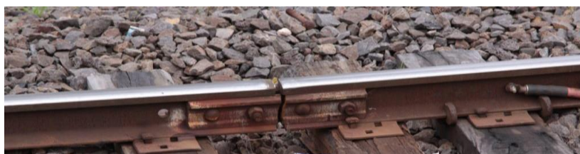
Figure 2.3: Railway track joint.
