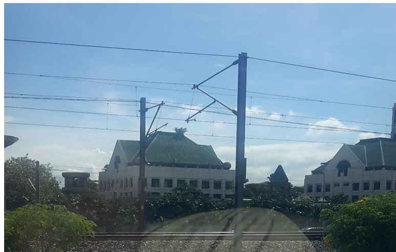
Figure 2.11: Railway track showing of MTLs in Malaysia
