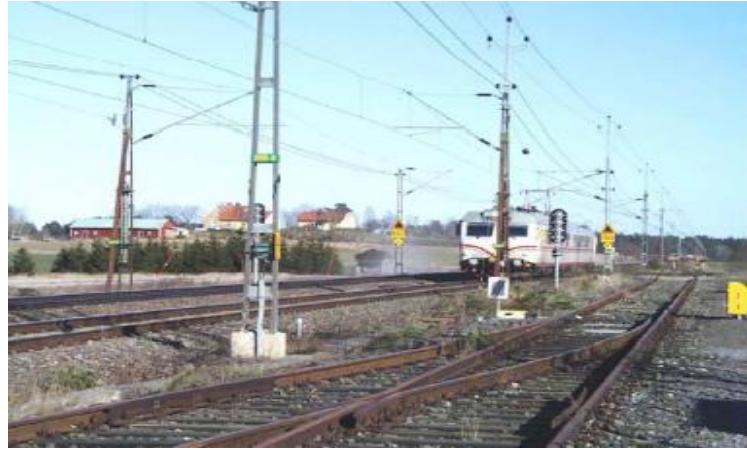
Figure 2.10: Railway track showing the complexity of MTLs.
