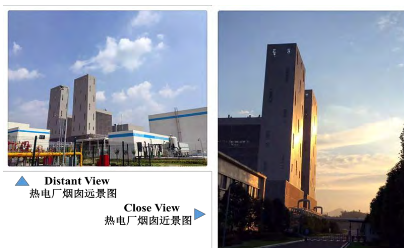
Fig. 3.9 On-site view of chimneys of thermal power plant
