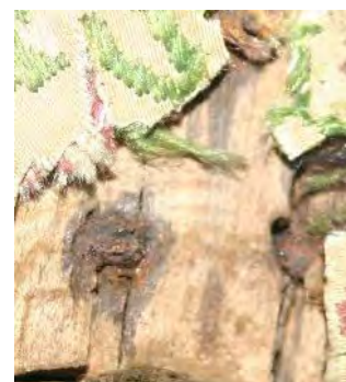
Figure 311 Corroded iron tacks causing splitting in wood. Clarks W17sD3 [11]
