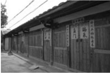
Fig. 10. Street interface of shoujinliao, Quanzhou
