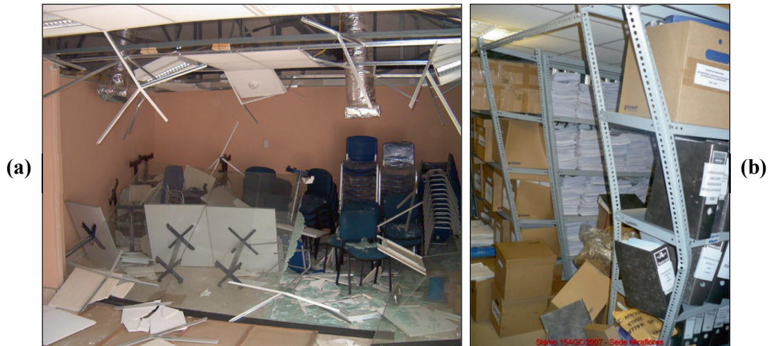
Fig.1 (a). Non-structural damage at the Customs Office a three-story R.C. building in Pisco city, Peru. Intensity VIII MMI. 1(b). Damage to contents in SUNAT, 14-story RC building in Lima, Peru. Both damaged by the Ica Region earthquake Mw 8.0 (USGS) of August 15, 2007.
