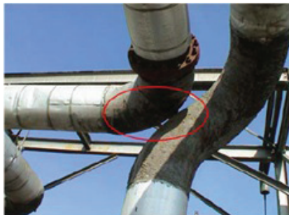
Figure 8: Adjacent Pipelines are vulnerable due to interaction effects
