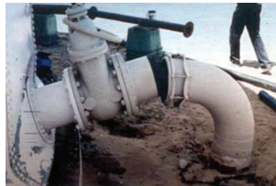
Figure 6: Unanchored Flat Bottom tank Slides and Rocks (ALA 2002)
