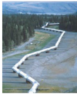
Figure 3: TAPS pipeline and supports
