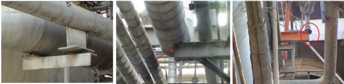
Figure 9: Inappropriate Supports
