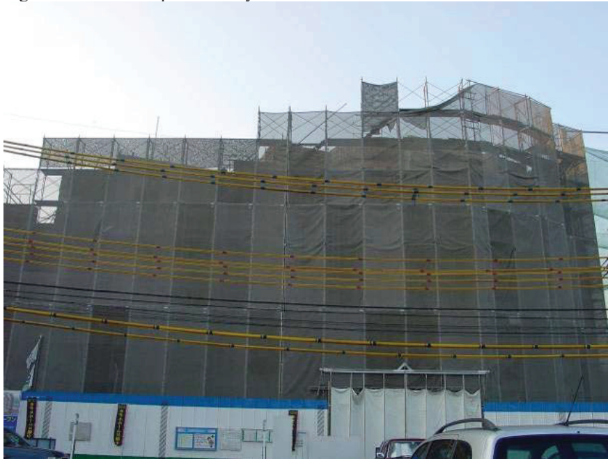
Photo 1: Scaffolds covered with sheeting.
