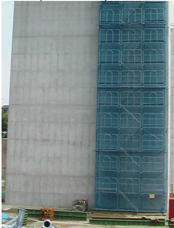
Photo 3: Prefabricated scaffolds constructed by guardrail-first erection method.
