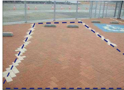
Fig. 10. Application to paving blocks
