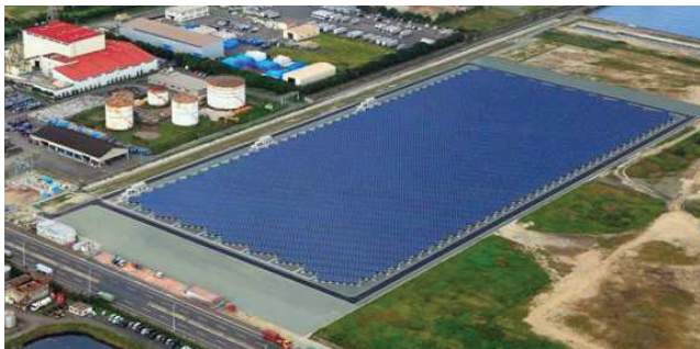
Fig. 7. FUKUYAMA Photovoltaic Power Station
