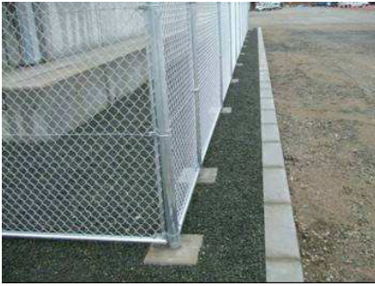
Fig. 9. Application to foundation blocks
