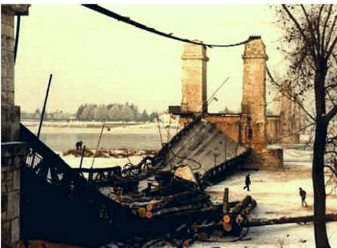
Fig. 2. Bridge collapse in Sully-sur-Loire (January 1986) due to a truck accident.
