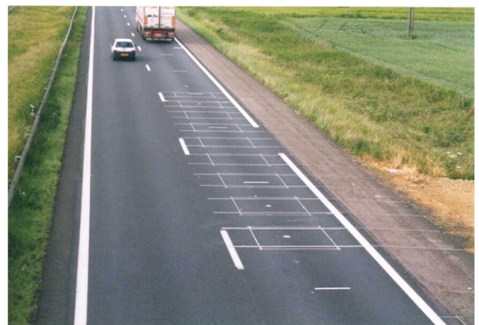
Fig. 7. MS-WIM (multiple sensor) array on the A31 motorway (East of France).
