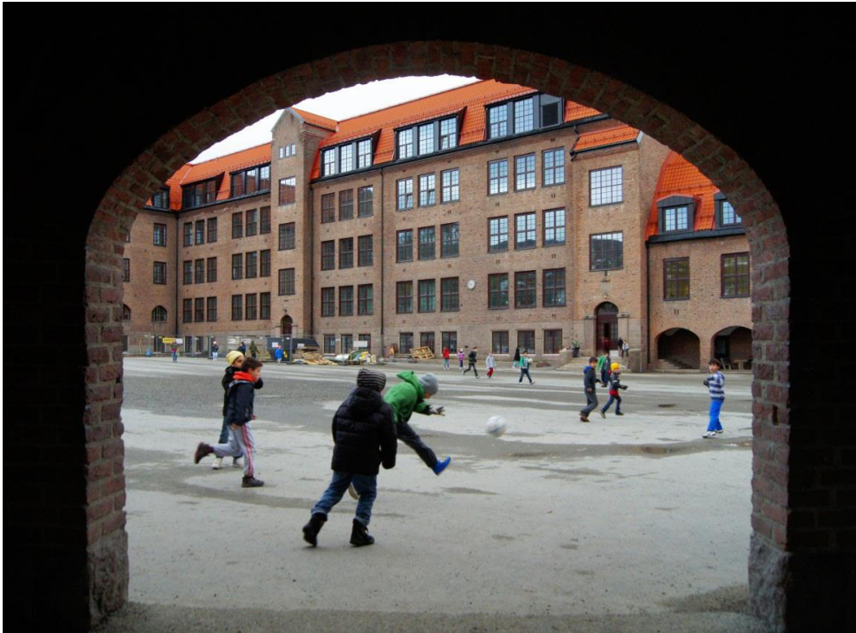
Fig. 5. South façade after replacement of windows and roof cladding. Photo: S. Røgeberg, Mai 2012. Architect for the retrofitting: a-form architects / Nils Herland.
