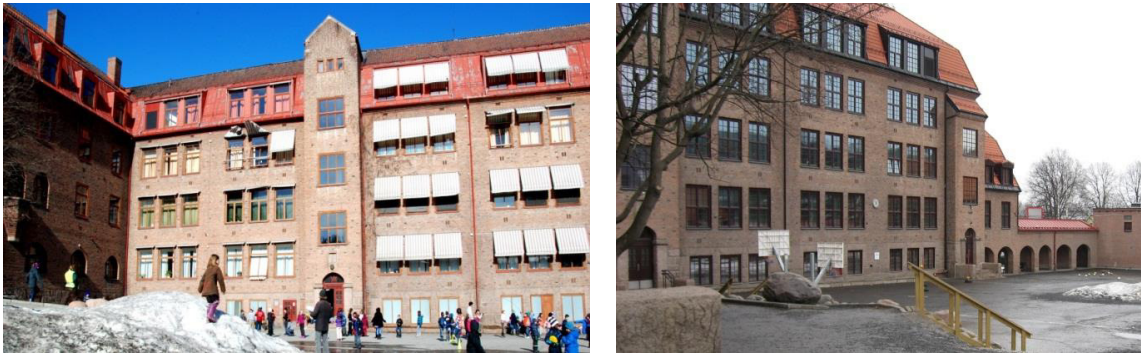
Fig. 2. (a) South façade before retrofitting; (b) South façade with new windows and roof cladding.
