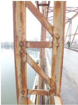
Fig. 2. Surface corrosion
