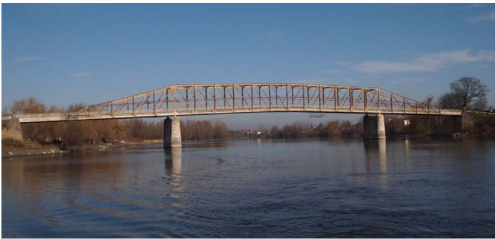
Fig. 1. Appearance of road steel bridge in Morovic
