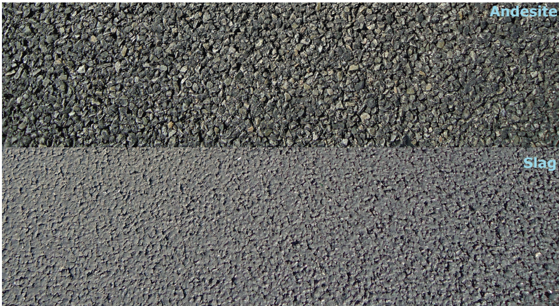
Fig. 4. Surfacing with natural aggregate of andesitic origin (top) and slag (bottom)
