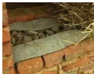
Figure 5 Moistureproofing method for straw-bale wall at the foundation.
