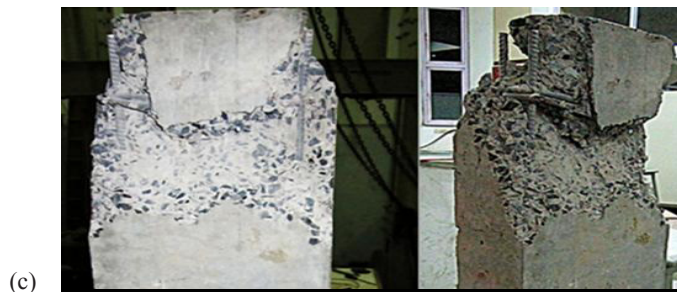
Fig.11 (c) Control rectangular column
