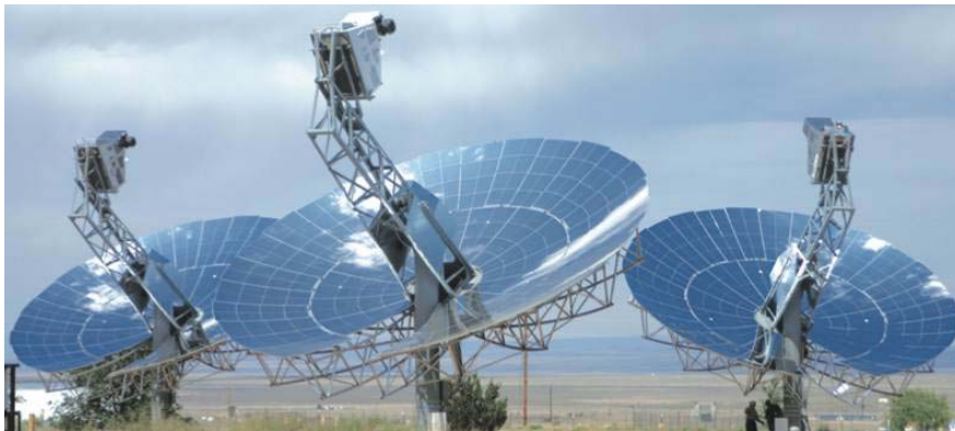
Fig. 1. Solar dish Stirling engine system [6]
