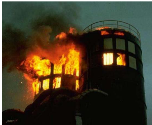
Fig. 7. Flames emerging from vent openings after a dust explosion.
