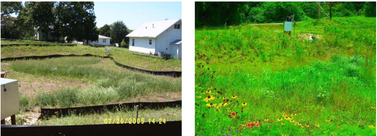
Fig. 2. Quinton Heights site after planting in July 2005 and at the beginning of the third growing season in May 2007. Note the grassed waterway through the bottom of the cell was planted with prairie cord grass plugs while the rest of the site was drilled with seed
