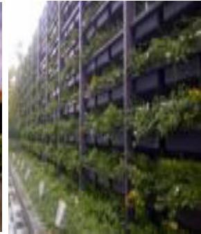
Fig 7. Intermark Integra Tower Source: Author's archive (2013)
