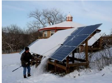
Fig. 1. Clearing of accumulated snow off PV modules [1]
