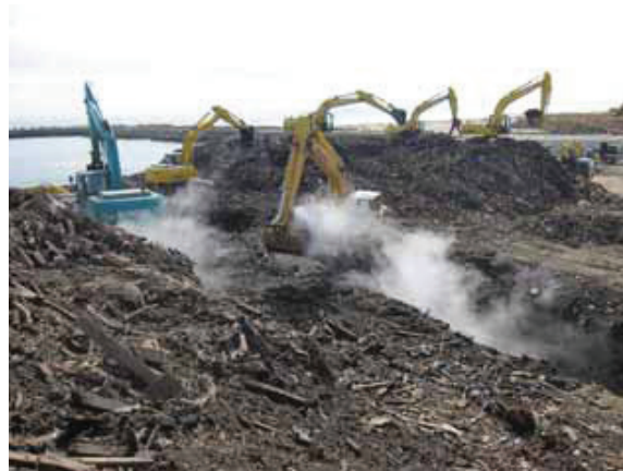
Fig. 1. A picture of rubble pile. During dealing with rubble, huge smoke and water vapor was produced and temperature of surface of materials are high, at least 60°C.
