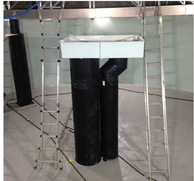
Fig. 6. Large drain structures used to rapidly remove dead or moribund fish from the tank center provide a huge benefit to the tank operator but also impact culture volume hydraulics.
