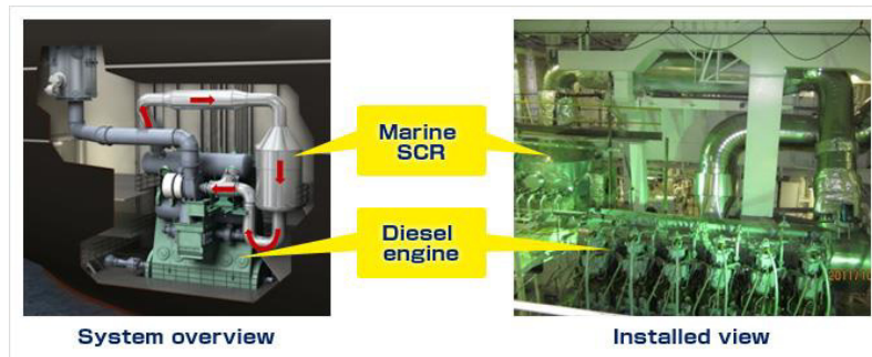
Fig. 2. Marine SCR system (Hitachi Zosen Corporation ).
