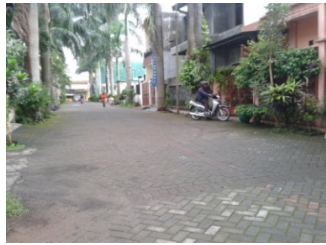
Fig. 5. Physical condition of segment B2
