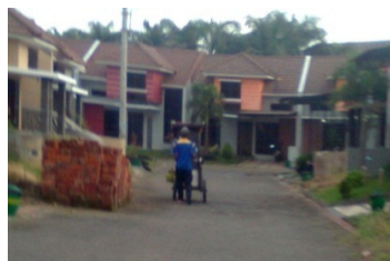
Fig. 4. Physical condition of segment B1
