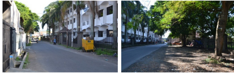
Fig. 3. Physical condition of segment A3
