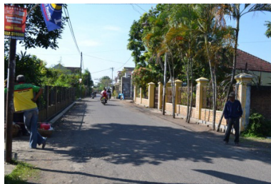
Fig. 7. Physical condition of segment C1
