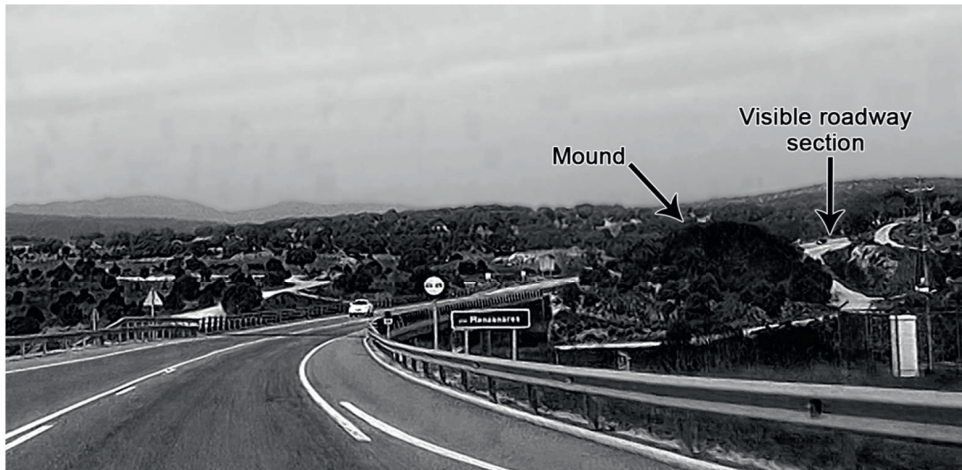
Fig. 2. Mound causing a hidden section and visible roadway section beyond in M-607.
