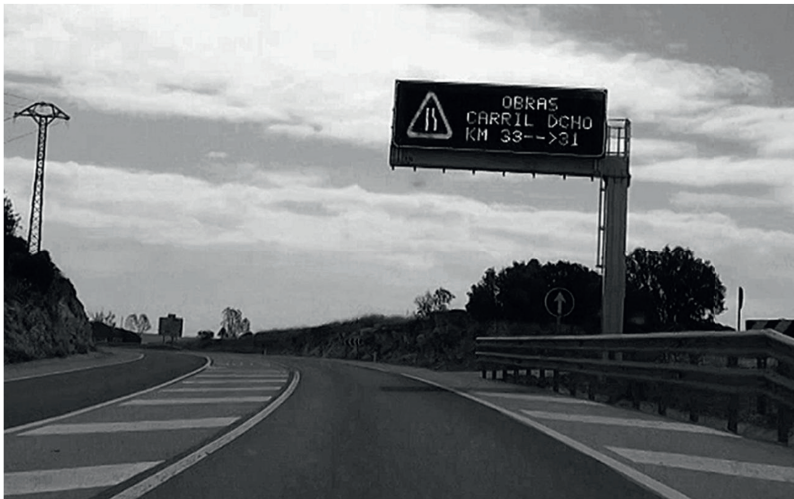
Fig. 4. Single-leg gantry signal in M-607.
