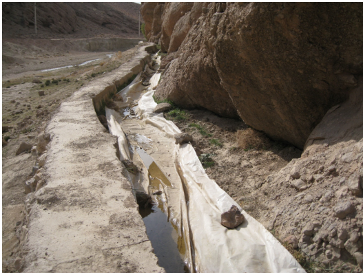
Fig. 3. Plastic cover to keep and convey the water
