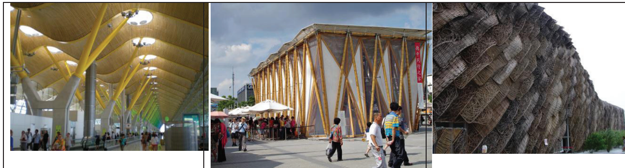
Figures 4, 5, 6. Upper right: Terminal (NAT) Barajas Airport (Madrid, Spain). Source: Photographs by the author. August 2011. Middle; German Chinese House. General view. Source: Photographs by the author. September 2010. Upper left: The Spanish Pavilion, made by rattan, wicker and bamboo. Source: Photographs by the author. September 2010.
