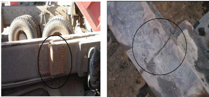
Figure 1 the fatigue crack of the sub-frame
