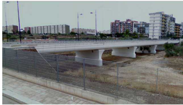
Fig. 4. View of the completed viaduct.
