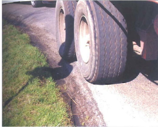
Figure 1. Edge loadings occurring on narrow traffic lanes.
