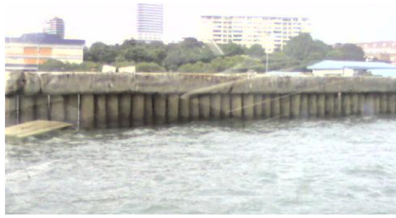
Fig. 1. A section of the pile breakwater next to Pasir Panjang, Singapore.
