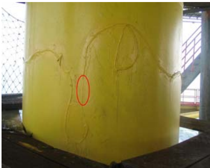
Fig. 2 FBG strain sensor installed on the pile leg
