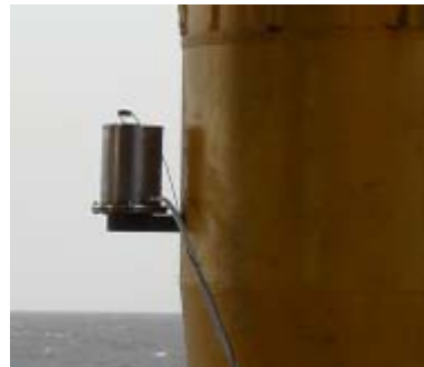
Fig. 3 Differential settlement monitoring equipment
