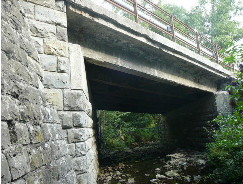
Fig. 11. Bridge superstructure - view.
