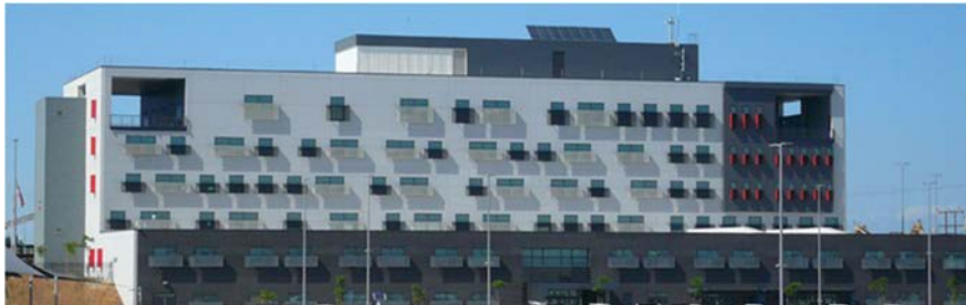
Fig. 3. Sacramento Municipal Utility District (SMUD) East Campus Operations Center, Sacramento, CA.
