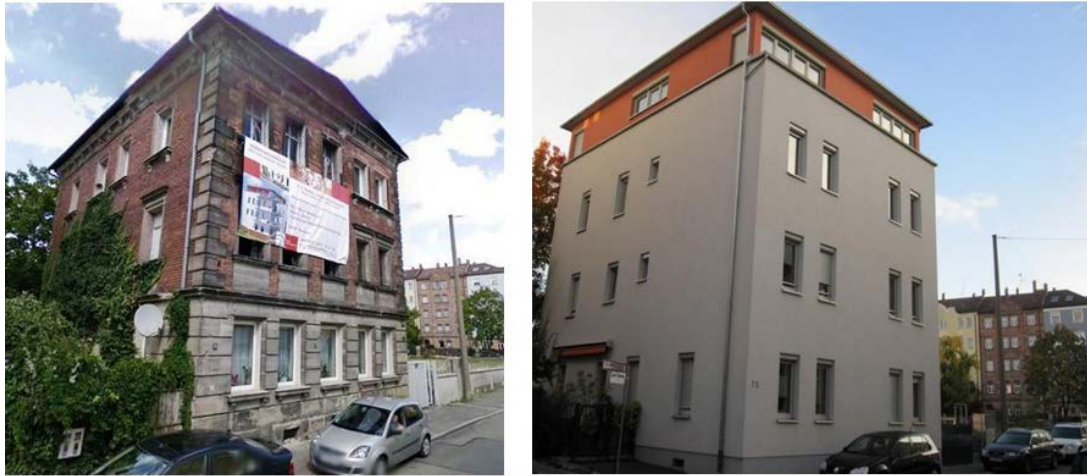
Fig. 1. Thermal insulation historical building, Ludwig Feuerbach-Strasse 75, 90489 Nuremberg Germany [3]
