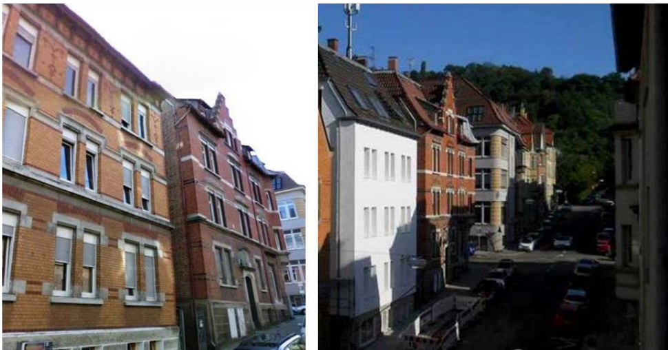
Fig. 2. Thermal insulation house in Stuttgart (Schreiberstraße 23), Germany [3]
