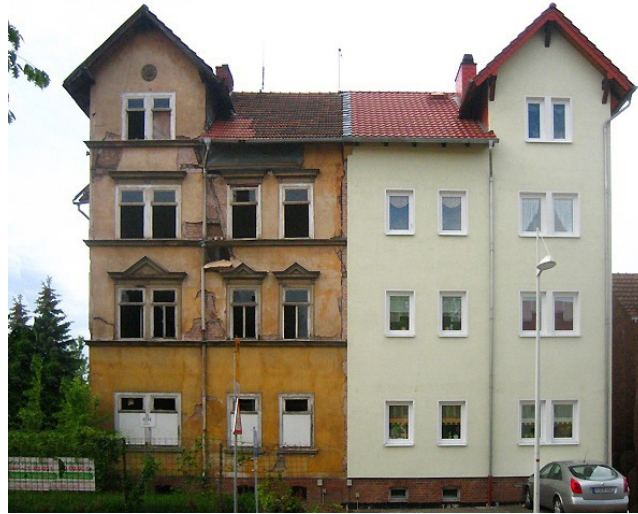
Fig. 3. Thermal insulation historical building in Eisenach, Germany [3]
