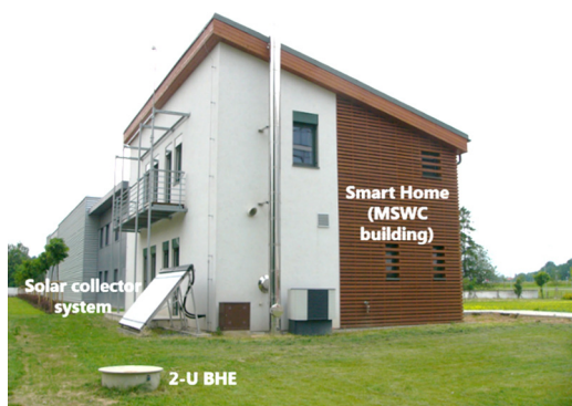
Figure 1 MSWC building – view on this smart one-floor wooden house and installed technologies (i.e. a 2-U borehole heat exchanger with the fifth pipe for measuring some uninfluenced/influenced temperature profiles, and the solar collector system).
