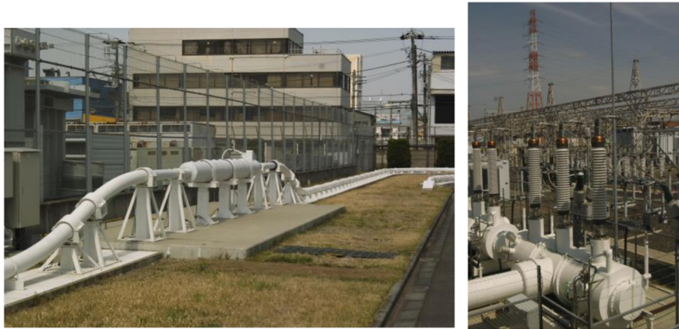
Fig. 2. TEPCO/Sumitomo 66 kV AC HTS test station at Asahi substation in Yokohama/Japan: left image shows the cable with a joint, right image shows the 66 kV AC end stations responsible for the transition from standard conductor to superconductor and from room to cryogenic temperature (2014).
