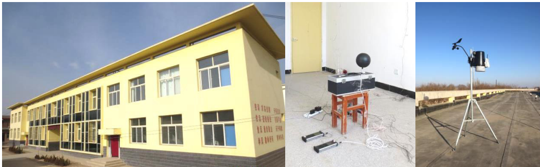
Fig. 1. Experimental building, measuring point of indoor and outdoor thermal environment.
