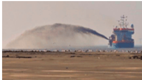
Figure 6. Spreading of sand slurry for land expansion purposes
