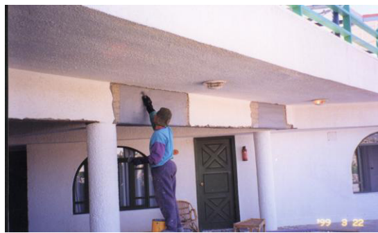
Figure 31. Surface preparation of beams
