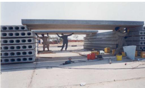
Figure 6. Prestressed slabs strengthened with FRP
