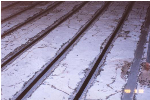
Figure 30. Flexural strengthening of slabs
