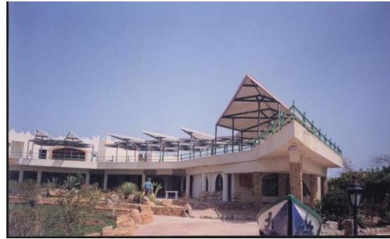
Figure 33. The Panorama building after retrofit
