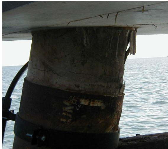
Figure 22. Concrete Crushing
