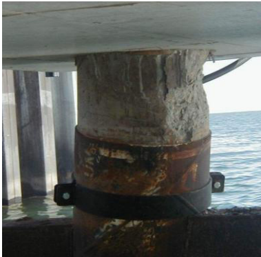
Figure 23. Removed concrete
