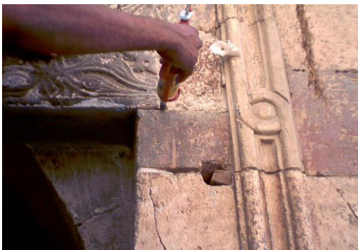
Figure 19. Holes at the ends of the lintel
