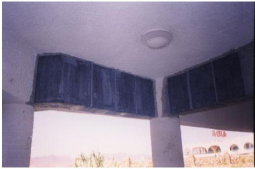
Figure 32. Shear strengthening of beams
