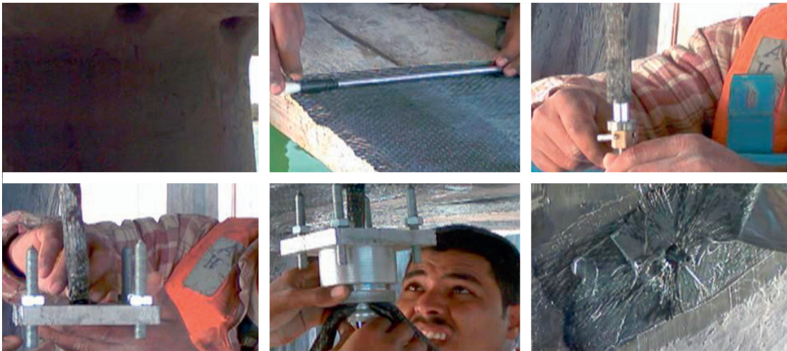
Figure 28. Applications of CFRP anchors
