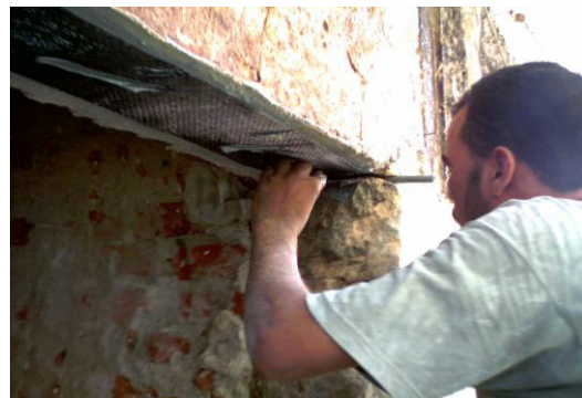
Figure 20. CFRP laminates at the bottom face
