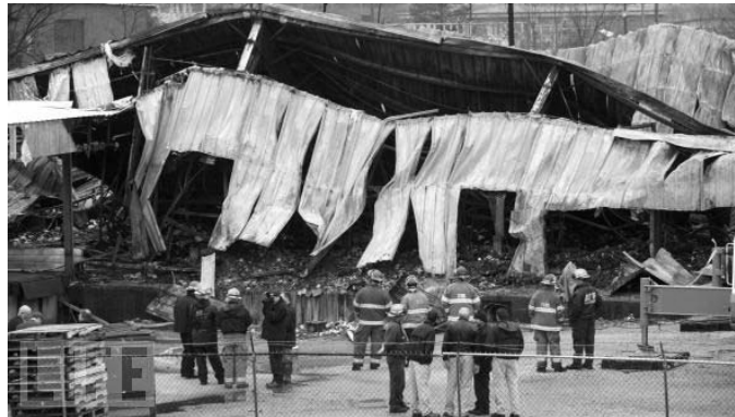
Figure 6: A collapsed portal frame structure
