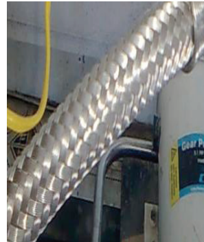
(b) Metallic flexible hoses unharmed at vacuum
