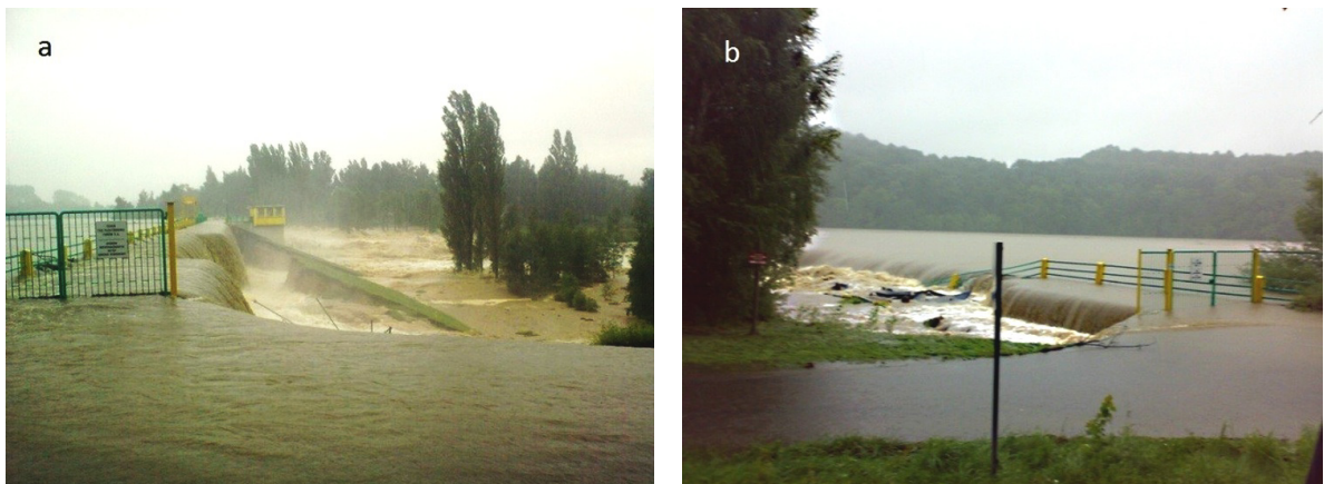
Fig. 3. Phase 2: (a) right side of the dam, 5:42 PM, water level H = 212.00 m a.s.l., (b) left side of the dam, 5:56 PM, H = 211.60 m a.s.l.
