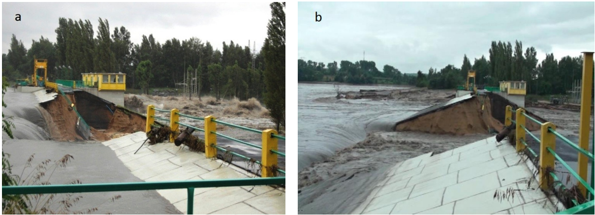
Fig.4. Phase 3 of the right side: (a) 6:22 PM, water level H = 210.70 m a.s.l.; (b) 7:45 PM, right side, empty reservoir.
