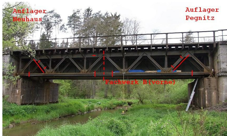
Fig. 1. Pegnitz railway bridge; locations of the strain gauges.
