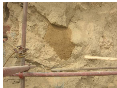
Fig.11 Anchor hole with completion of old treatment.
