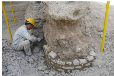
(a) During reinforcement.
