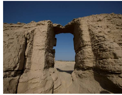
Fig.8 Doorway of the official building before and after consolidation.
