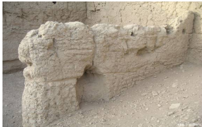
(b) After reinforcement.
