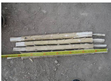
Fig.3 Wooden anchor employed for reinforcement of earthen site.
