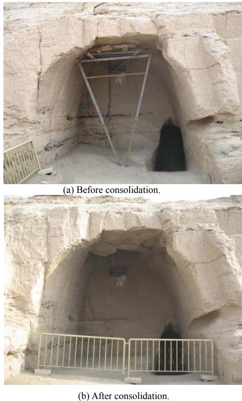
Fig.7 West cave opening of the official building before and after consolidation.
