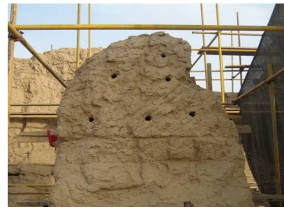
Fig.4 Pre-drilling anchor holes before sealing.
