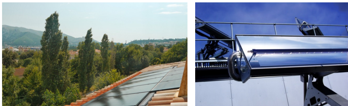
Fig. 2. A roof integrated PV/T system in Marseille, southern France (left, photo courtesy of DualSun), and the Absolicon PV/T installation to the local hospital in Härnösand (right, photo courtesy of Absolicon).
