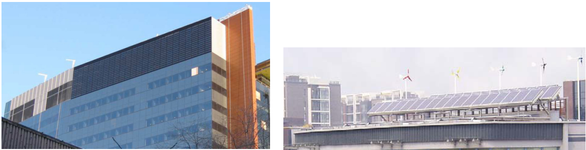
Fig. 1. The SolarWall PV/T facade at Concordia University, Montreal (left), and the SolarWall PV/T installation on the Olympic village in Beijing (right). SolarWall® PV/T system, photos courtesy of Conservall Engineering.
