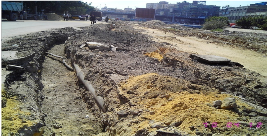
Figure 2 Example of electricity projects causing delays.
