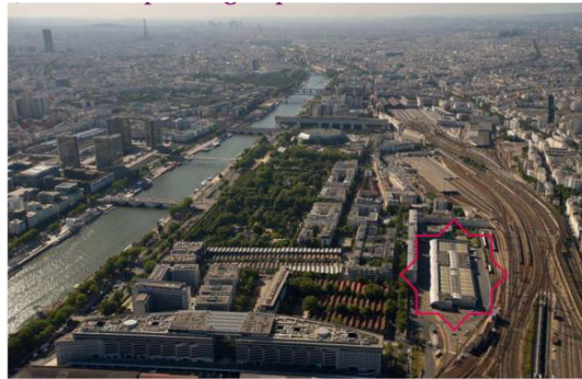
Fig. 2. Monoprix Samada rail terminal (Paris) (Source: Samada)
