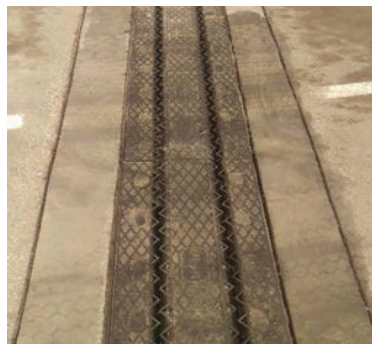
Fig. 12. Nezavisimosti Av. crosses Filimonova str. (expansion joint installed in 2015).
