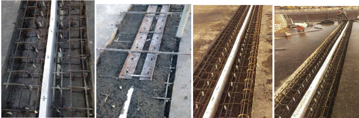
Fig. 9. Expansion joint structure with a rubber compensator with traffic preserved next to it. High-strength concrete was used.
